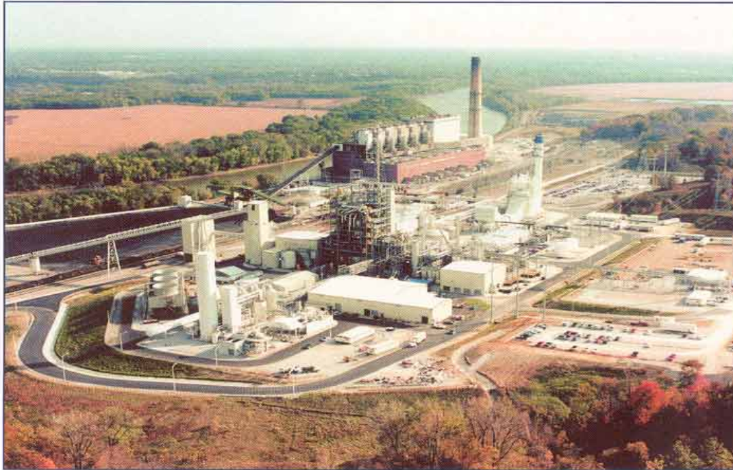
The Wabash River Coal Gasification Repowering Project
